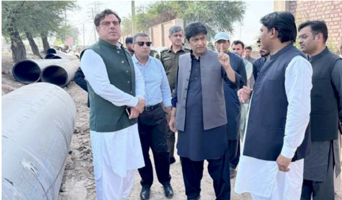
According to the briefing, projects worth Rs25.8 billion are currently underway in Multan city alone. These include the laying of 232 kilometres of RCC sewer pipelines and 16 kilometres of HDPE force mains, along with the installation of 88 pumps, 41 generators and 40 transformers. In addition, modern machinery such as dewatering units, winch machines and excavators is being introduced to improve response capacity and ensure sustainable drainage management. Senior officials, including RPO Usman Gondal, Deputy Commissioner Noman Siddique and CPO Sadiq Dogar, as well as political representatives, attended the meeting.
